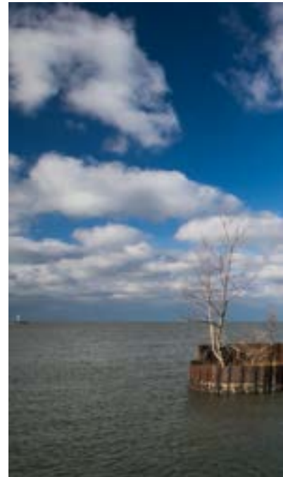
➤ Breakwater in front of the former FirstEnergy site (Cleveland Metroparks)
