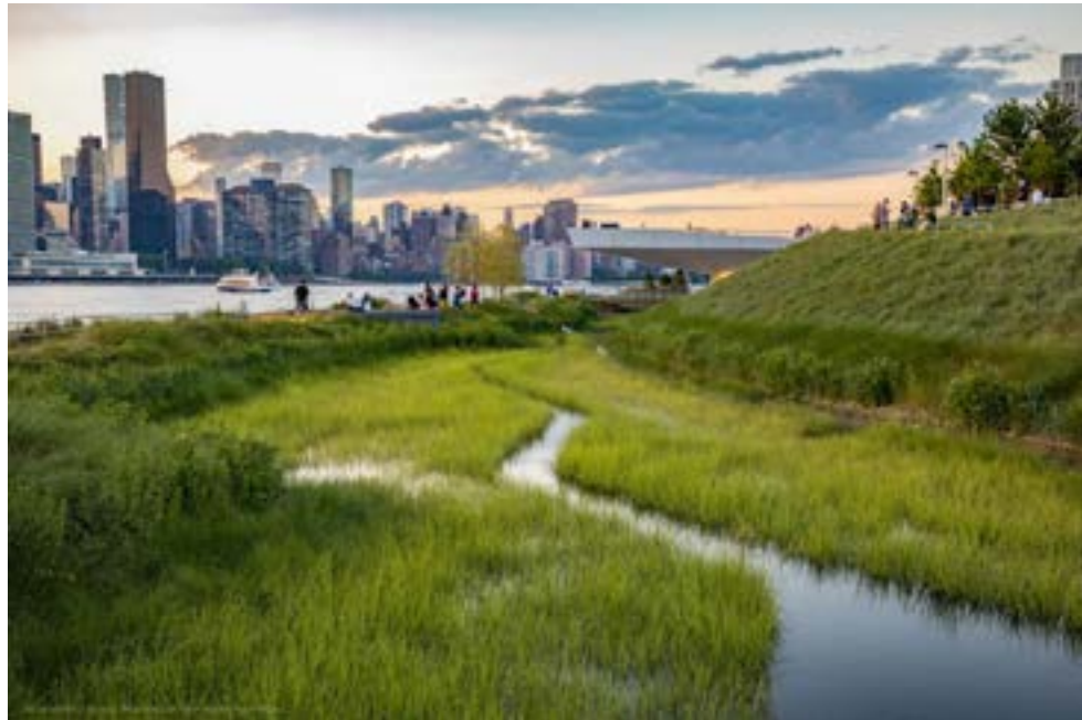
Figure 4: Example of riprap revetment and protected wetland habitat (source: SWA/Balsley n.d.)
