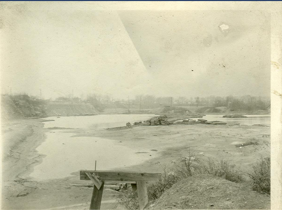
BEREA QUARRIES LOOKING NORTH #73
