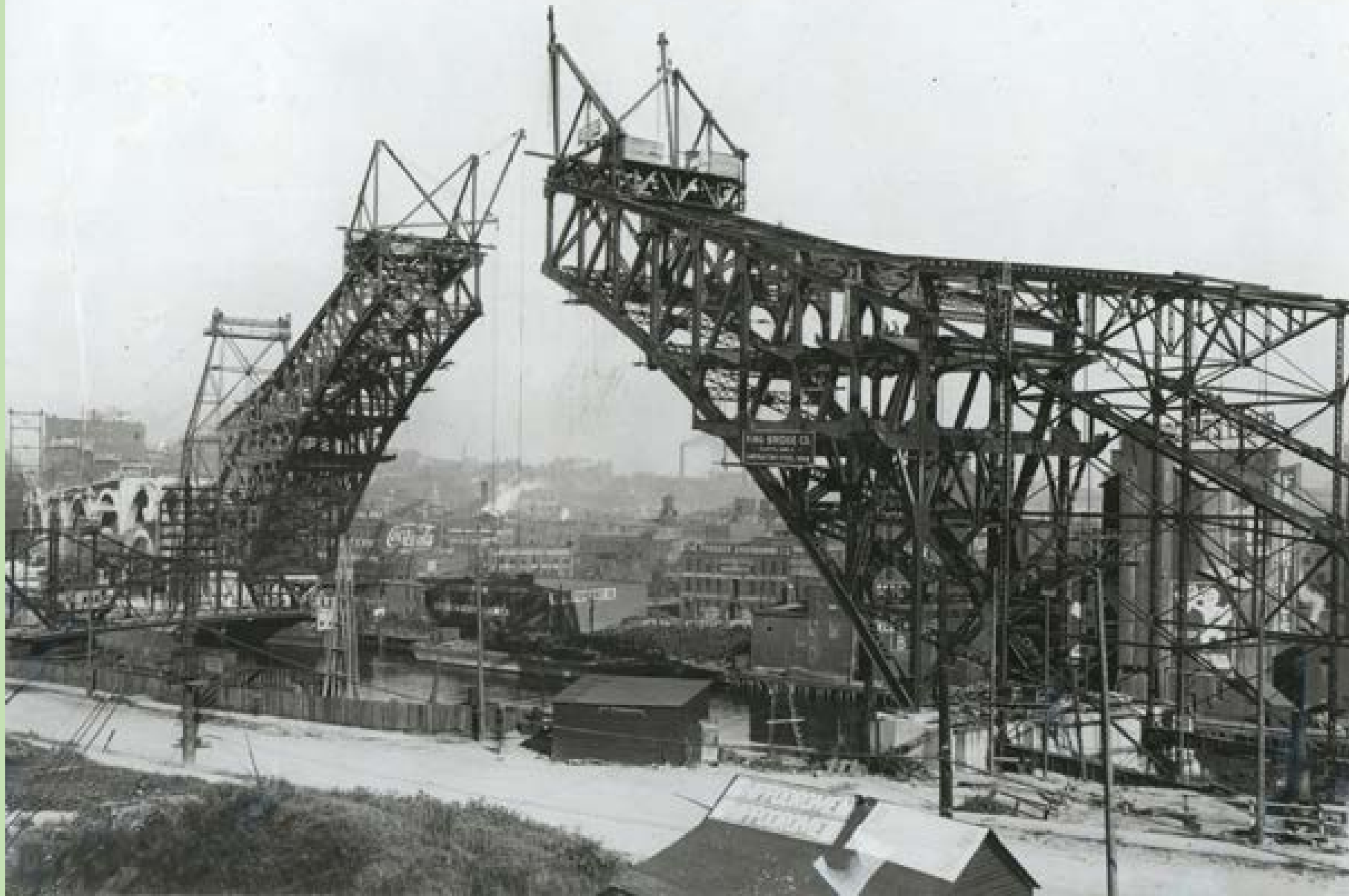
Construction of Detroit-Superior Bridge September 29, 1915
